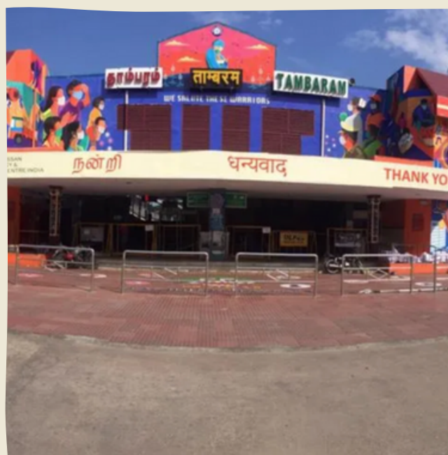
Tambaram Railway station
