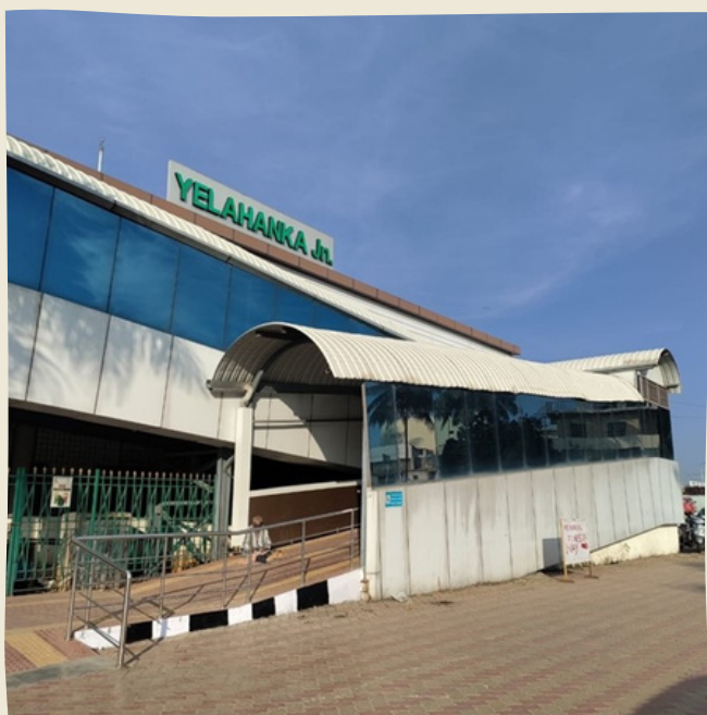
Yelahanka Railway station
