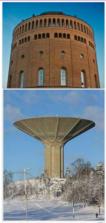
The mushroom-shaped concrete water tower of Roihuvuori in Helsinki, Finland was built in the 1970s. It is 52 metres high and can hold around 12,000 m<sup>3</sup> of water.
